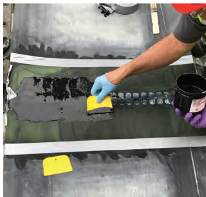
Before Metal Clips Splice Repair
